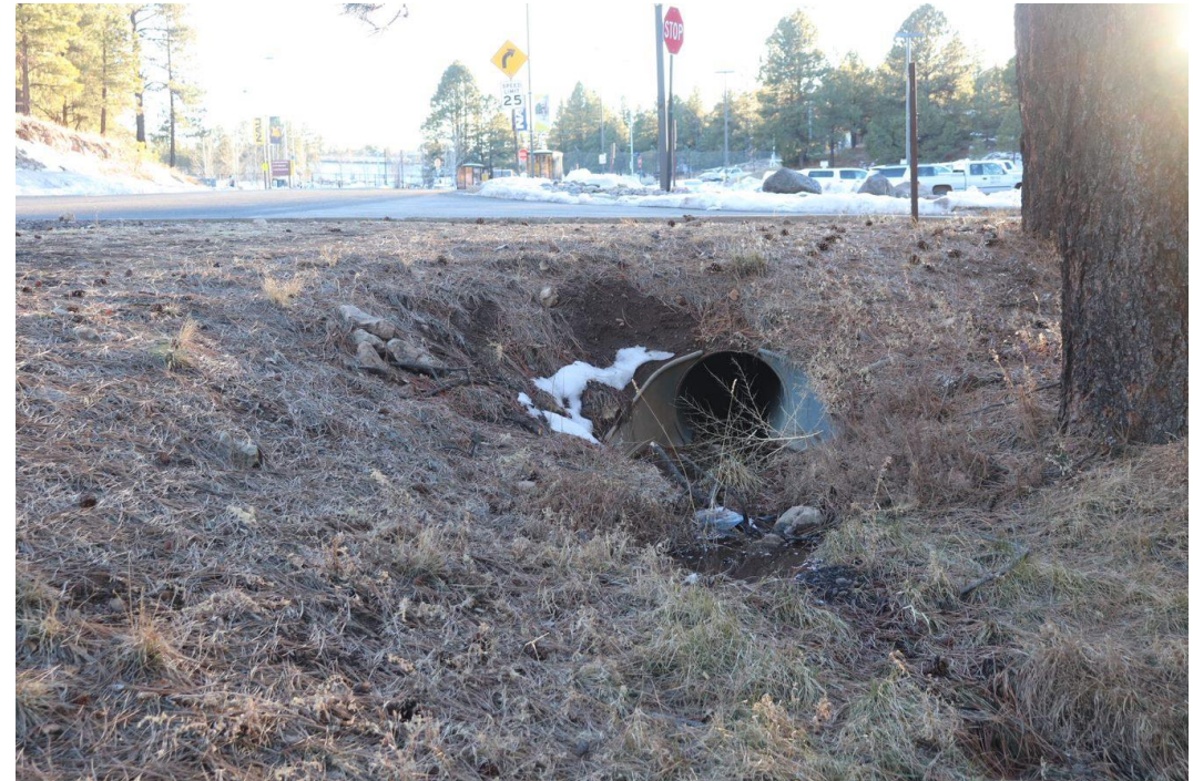
Figure 1-8: Culvert Outlet on South East Entrance of Parkinglot, Credit: Sophia Fox
