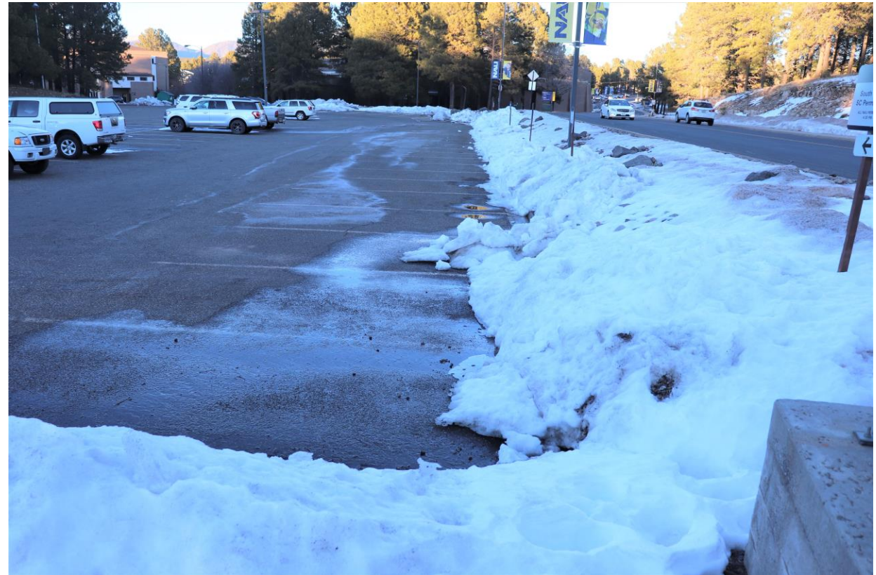
Figure 1-5: Southwest Corner of Parking Lot 46, Credit: Sophia Fox
